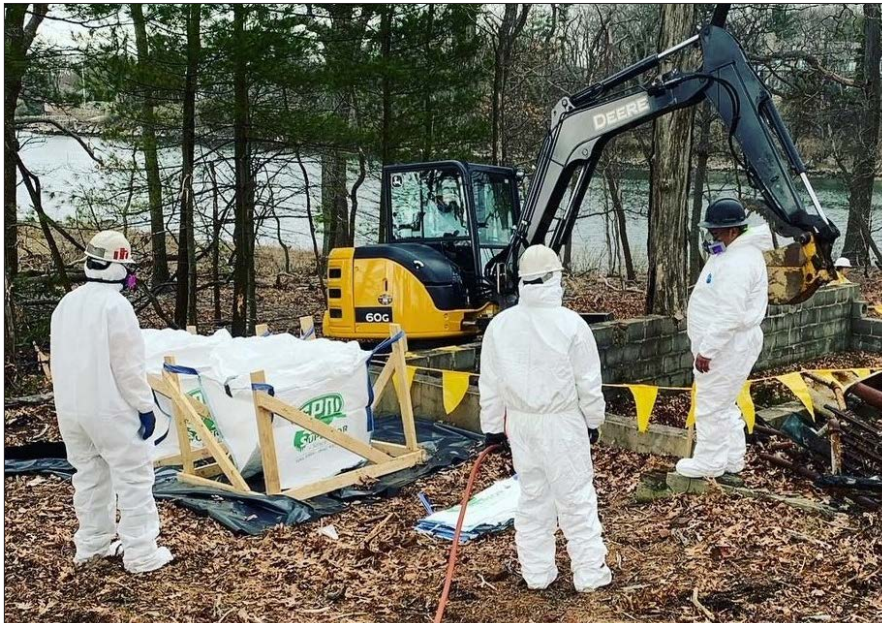
Environmental remediation contractors working under HRT Associates wear hazmat suits to protect from toxic PCBs and asbestos on Hoyt Island.
